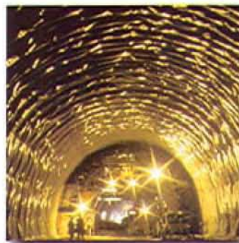
Sinber Tunnel in Austria. Carbofol®, with a damage indication layer, as a tunnel liner for moisture protection.
