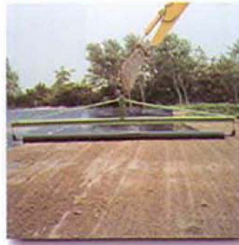
9.40 m wide Carbofol® as one part of a composite base seal.
